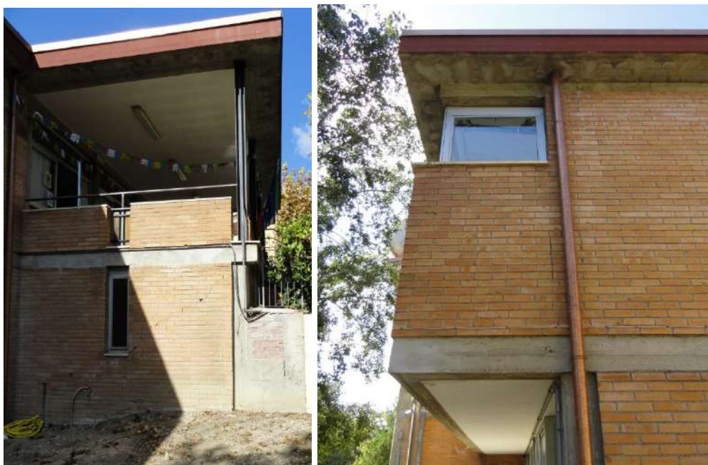
Figura: Vista gronde e velette in c.a. (lotto II)
